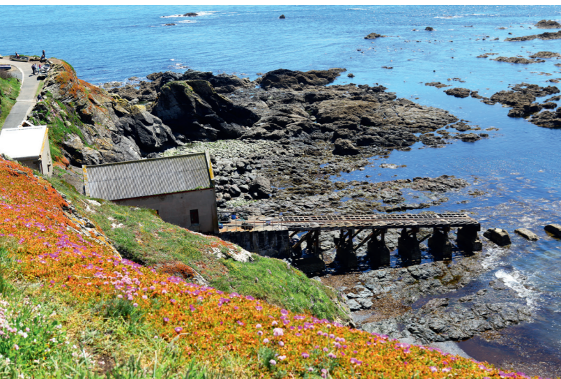
▲ The now-abandoned Lifeboat Station at Lizard Point
